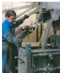
Lower heat exchanger, being cast into the refractory cement.
